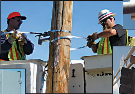
Mast Arm Sign Installation
