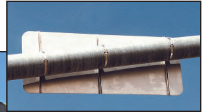
Mast Arm Sign Installation
